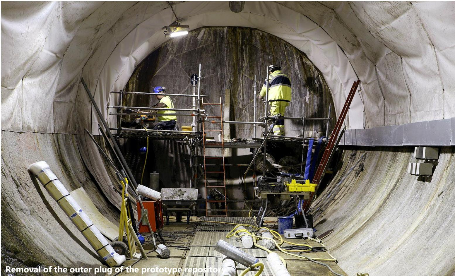
Removal of the outer plug of the prototype repository
